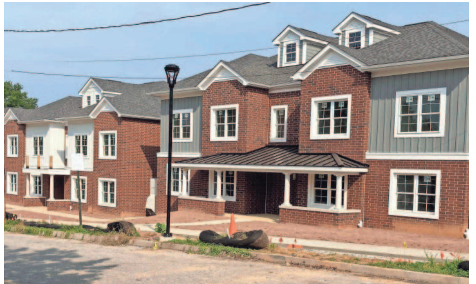
Nearing completion, the new streetscape in the 200 block of W. Springettsbury Avenue is York College-owned apartments available for upperclassmen. The buildings wrap around to Manor Street. SUBMITTED
